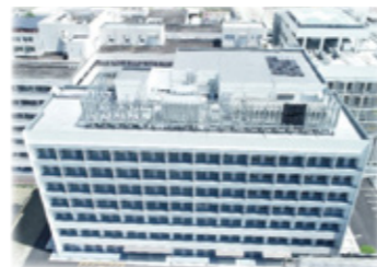
[Completed Second Stage Bldg.]
