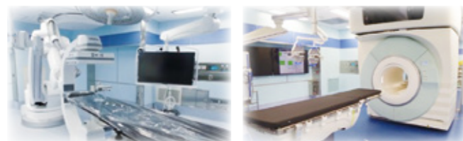
[Hybrid operating room]
