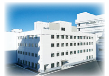
[ Completed Clinical Support Bldg.]
